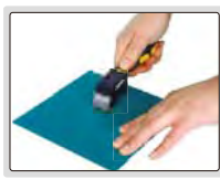
step 1: make grid cutting on surface
